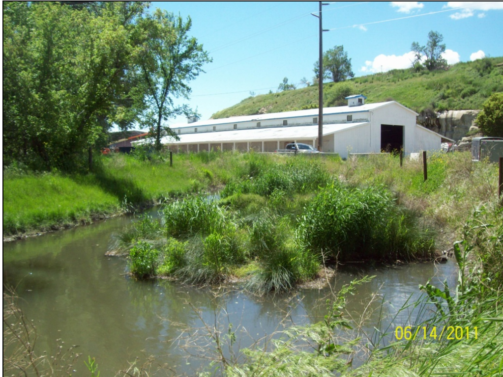
Metra stormwater pond with FTW, June 2011
