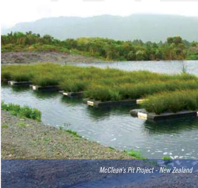
Effluent water - McClellan's Pit Project, New Zealand. Before and after treatment by BioHaven® floating treatment wetlands.
