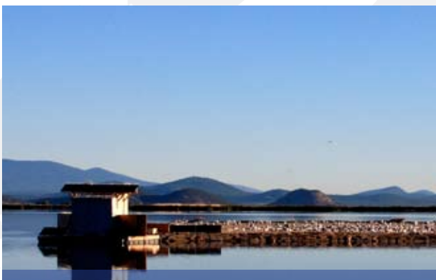
39,700 Ft 2 Sheepy Lake Caspian Tern Rookery, Army Corp of Engineers Project
