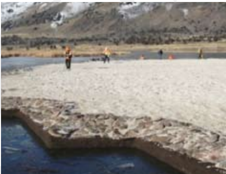
Completing the floating island - Dutchy Lake, Oregon
