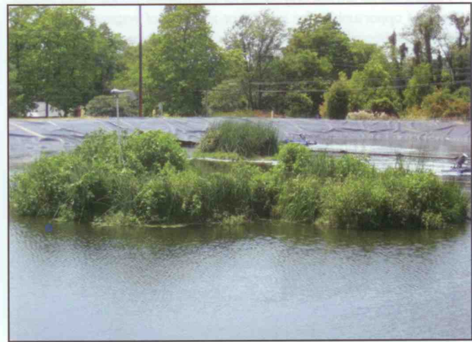
Wiconisco water treatment facility in Wisconsin, USA
