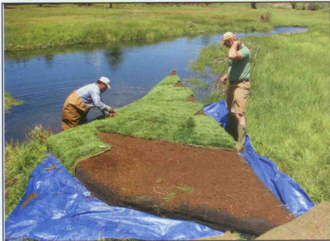
Islands being prepared for bank stabilisation
