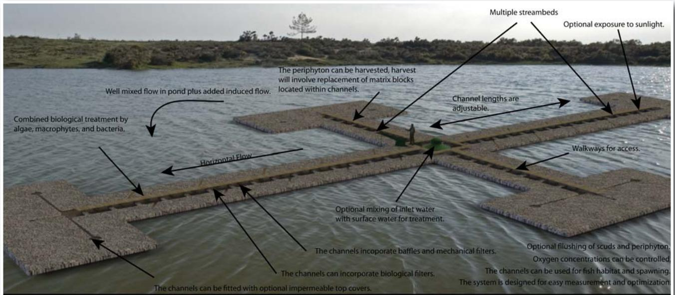
Figure 2. Schematic of Leviathan floating treatment wetland.
