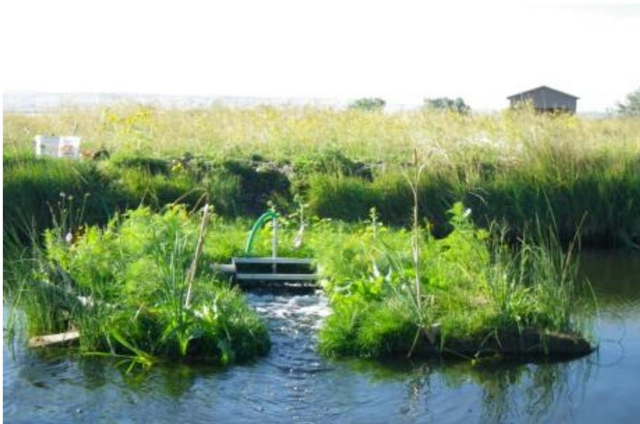
*The circulation generated by this small floating streambed's airlift system provides critical aeration in Minnow Pond's high oxygen demand environment*
